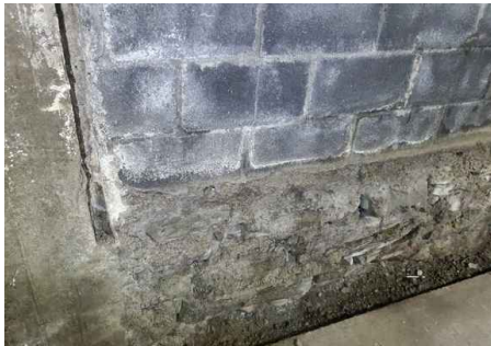
Original stacked stone with masonry block retrofit repair.
