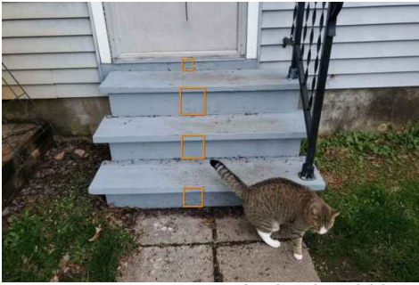
Stir risers are over 8.5" high. Should be between 7 and 7-3/8"
